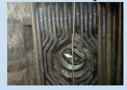
> D Type boiler panel wall retubing
